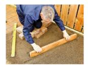
The laying course is normally a natural clean sharp gritty sand, laid moist in a 30–50mm layer and screeded off to correct levels. Alternatively, a clean grit may be used.
