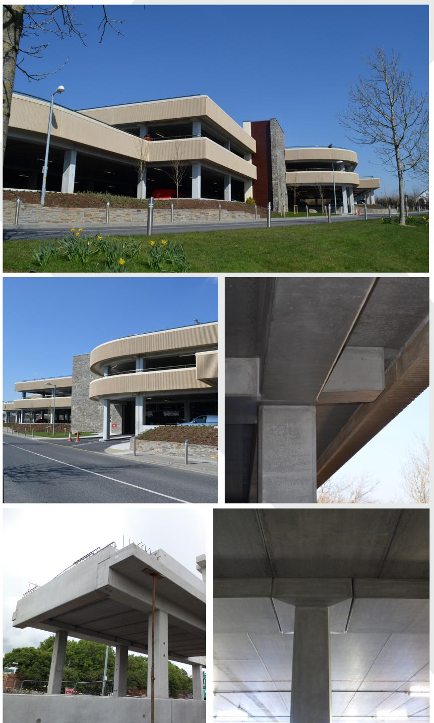
This project consisted of a fully precast 2 storey concrete frame solution. The beam and column frame was designed to cater for a future 2 storey vertical extension. There was a number of complex features involved in this project from design and manufacture viewpoints:
