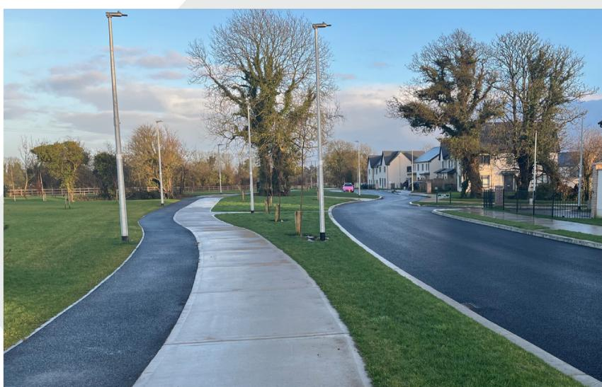
A Glenvegah residential development completed in 2023, Kilsaran Road Surfacing provided full access road and cycle track asphalt build up laying SMA10 PMB, AC20 Binder course and Ac32 Base course. The asphalt was produced using both RAP (reclaimed asphalt Pavement) and Thermaphalt (warm mix) resulting in a reduction in CO2 emmissions and conservation of aggregate.
