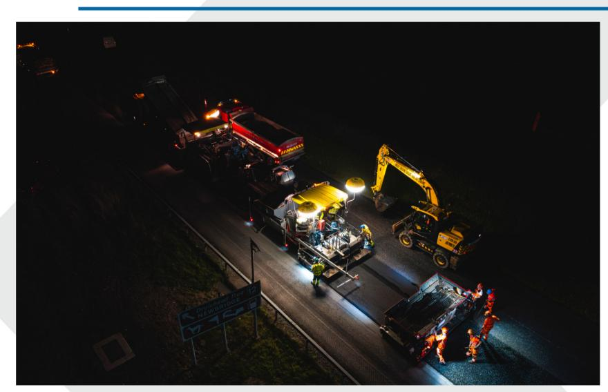
Kilsaran resurfaced 12km of carriageway on the M7 Kildare bypass pavement scheme for Jons Civil Engineering Limited. This was completed using 15,000 tonnes of Hot Rolled Asphalt (HRA) incorporating 15% RAP (recycled asphalt) The use of 15% RAP in the HRA materials results in a reduction of 165 tonnes of CO₂ when compared with standard HRA. The overall project achieved a 21% reduction in carbon emissions.
